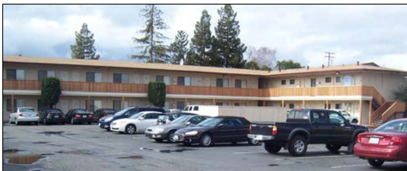
The newly remodeled St. Clare Housing.
