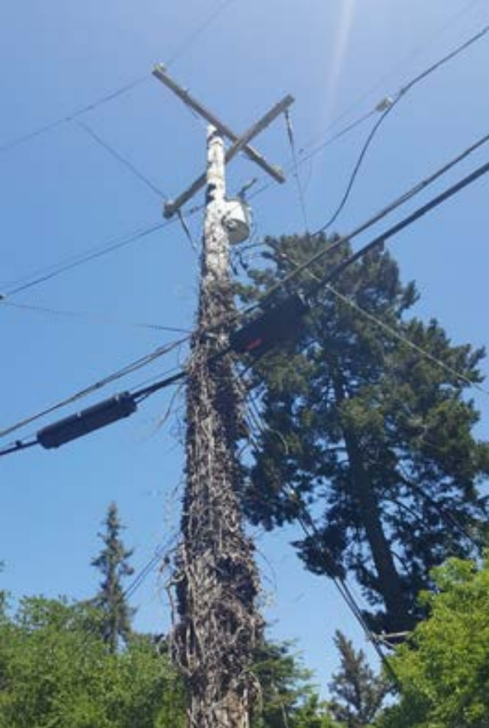
Photo: Tier 3 High Wildfire Danger Area, Los Gatos, CA, Utility pole wrapped with dead vegetation, Photo by Prof. Catherine Sandoval, May 2019
