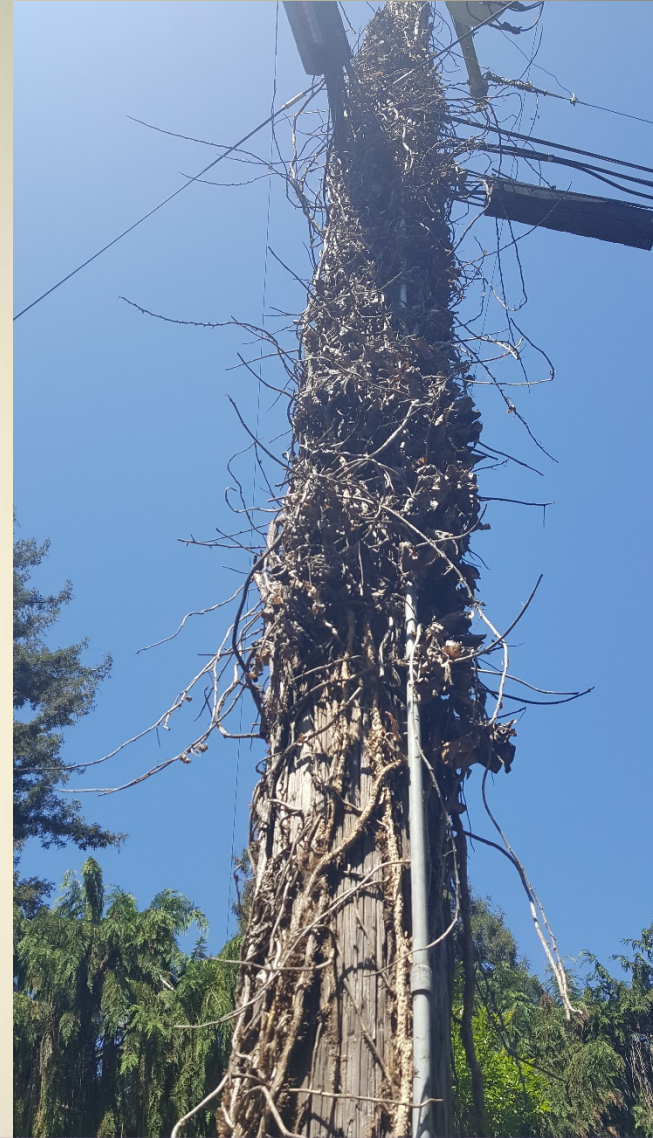
Tier 3 High Wildfire Danger Area, Los Gatos, CA, Utility pole wrapped with dead vegetation, photo by Prof. Catherine Sandoval, May 2019
